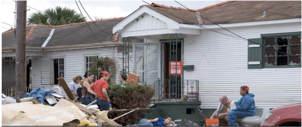
Cornell students emptied & gutted houses during January and March service trips
