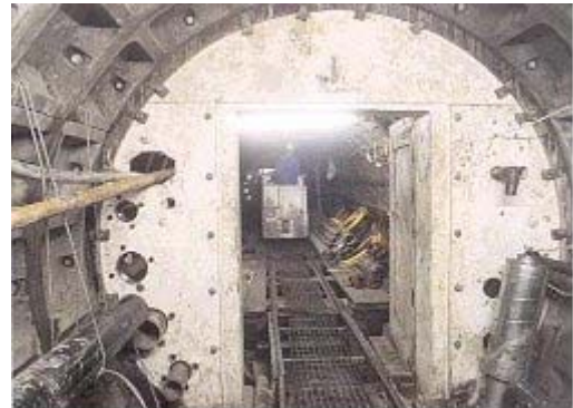
Northern Drainage tunnelling in progress
