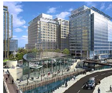
Churchill Place Development, Canary Wharf
